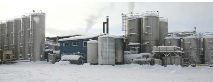
At the Alaskan Brewing Company, weather factors into plant operations.
